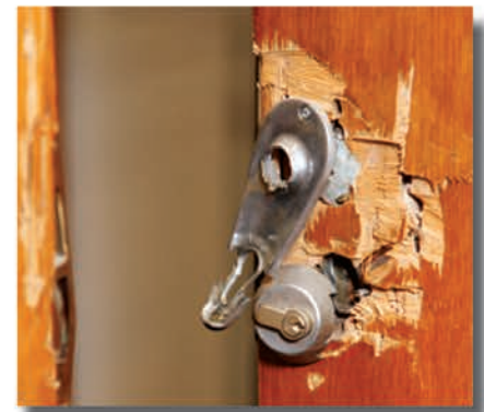
Home is Vandalized
